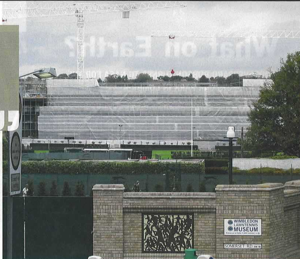
Match winner: Lytag concrete produced units 25% lighter than traditional concrete
