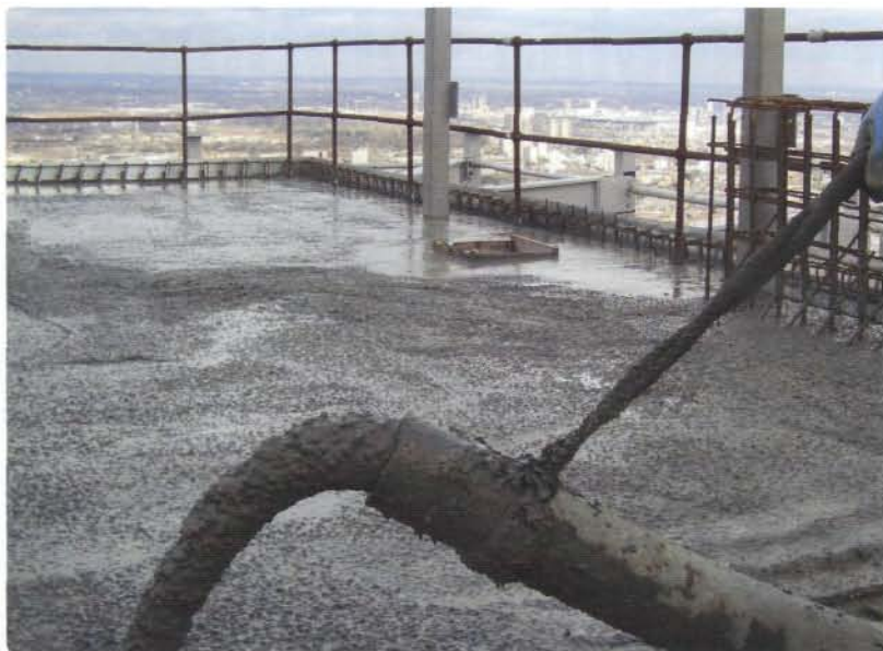
Pumping to the 41st floor of Heron Tower.
