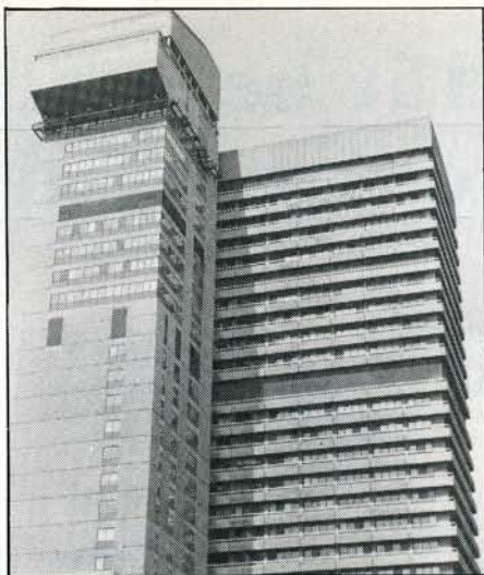
Figure 4: Guy's Hospital Tower near London Bridge Station, all the in situ concrete uses lightweight aggregate. Designed by R Travers Morgan and Partners
