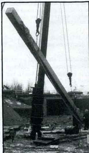
Amsterdam, Netherlands. pile being lifted into position before driving.
