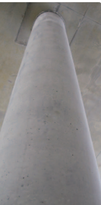
Figure 4: Fair-faced column in dining area.
