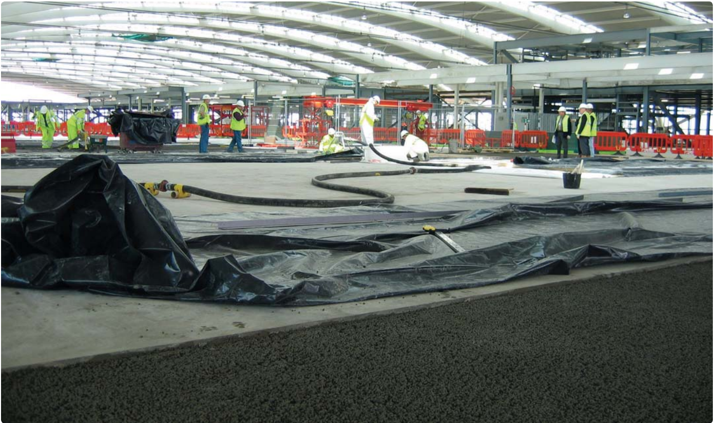
Figure 3: Upper floor of T5 during construction.
