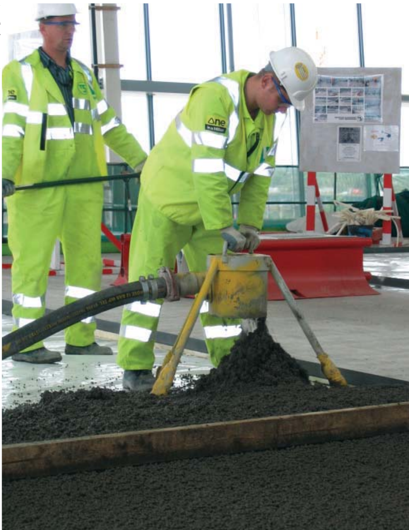
Figure 2 below right: Strip of placed Lytag no-fines screed.
