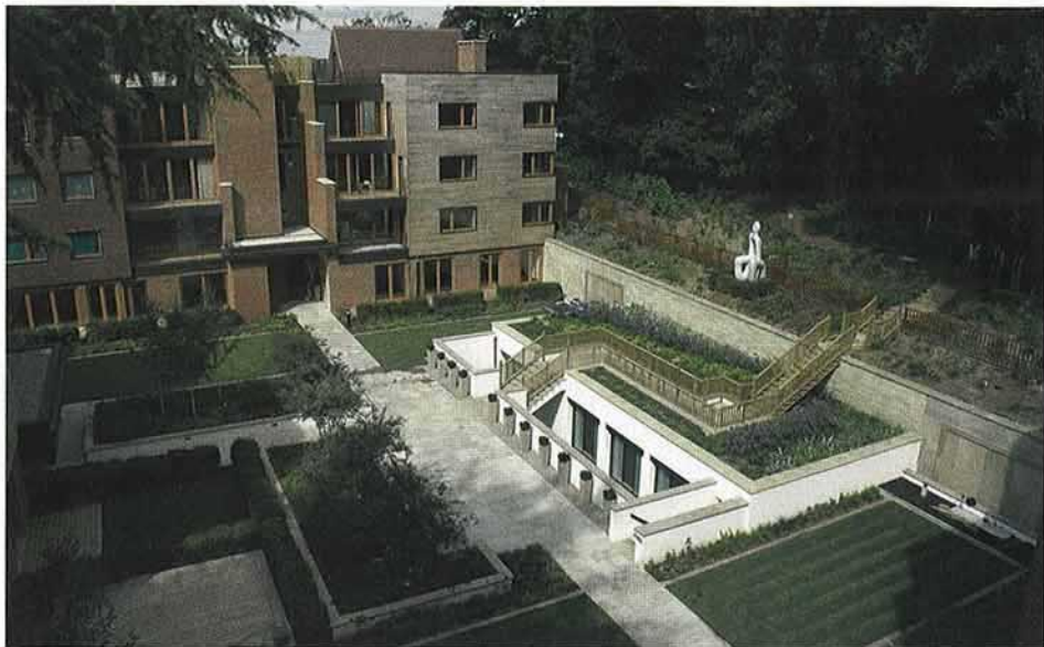
Living roofs incorporate the use of sustainable materials, support energy efficiency and provide a secondary drainage system.
