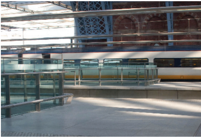
St Pancras Platform – lightweight no fines screed used to build up levels of the platform
