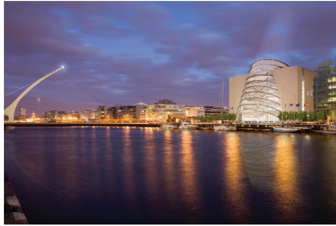
Samual Becket bridge and DCC – lightweight aggregate concrete used on the bridge deck to reduce loading and in the Dublin Convention Centre to reduce loading in the foyer main slab
