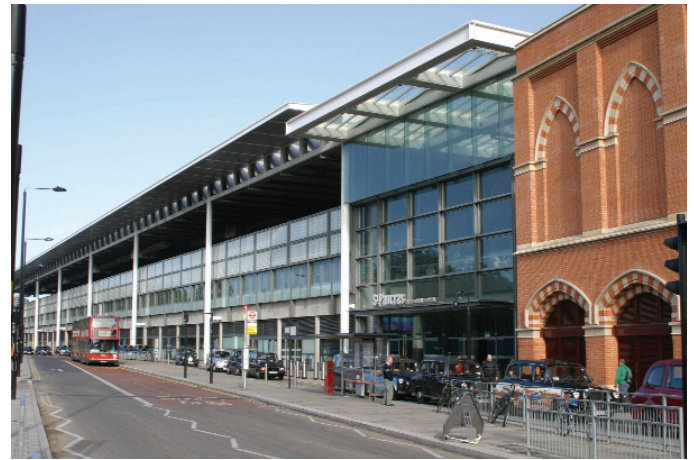
St Pancras Station – lightweight aggregate concrete used in the structure to reduce overall loadings in the structure
