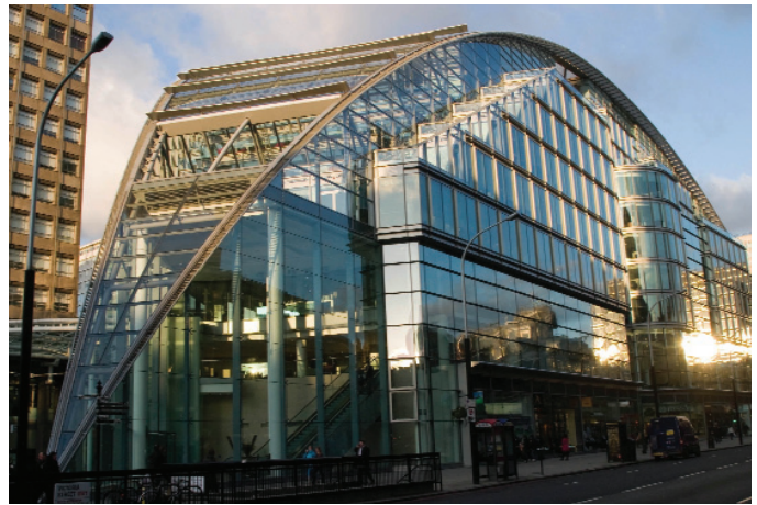
Cardinal Place, Victoria London – post tensioned lightweight aggregate concrete used to reduce overall loading within the structure
